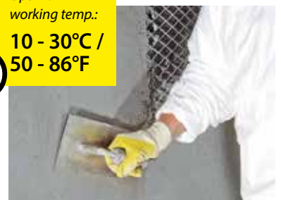
After spraying, easy to make smooth
