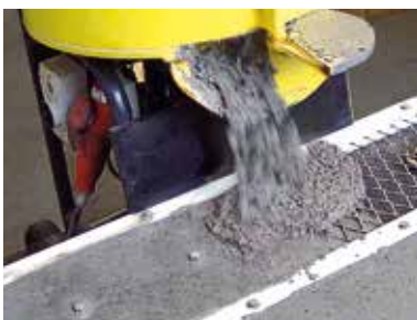
3. Carefully fill formwork
