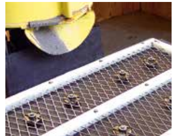
Prepare formwork, attach reinforcement system
