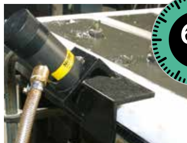
4. Use external vibrator for compacting
