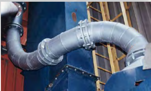
ABRESIST pipes and pipe bends protect against abrasion and corrosion
