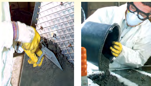
KALCRET can be installed by trowelling or casting
