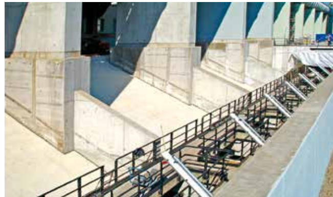
Kalenborn also successfully use KALCOR zirconium corundum and KALCRET hard compound in the area of coke loading bays
