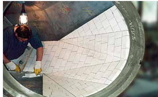
Octagonal hopper with KALOCER lining; for optimal adaptation the 50 mm thick shaped elements have been cut three-dimensionally
