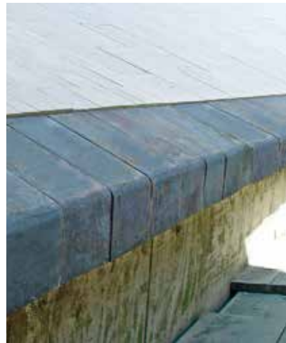
Kalenborn also successfully use KALCOR zirconium corundum and KALCRET hard compound in the area of coke loading bays
