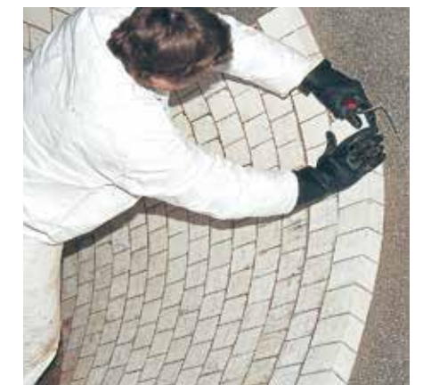
Kalenborn service solves wear problems on site
