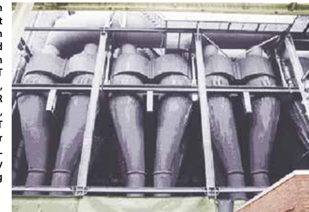
Dust collection cyclones for blast furnaces are effectively protected with combined linings
