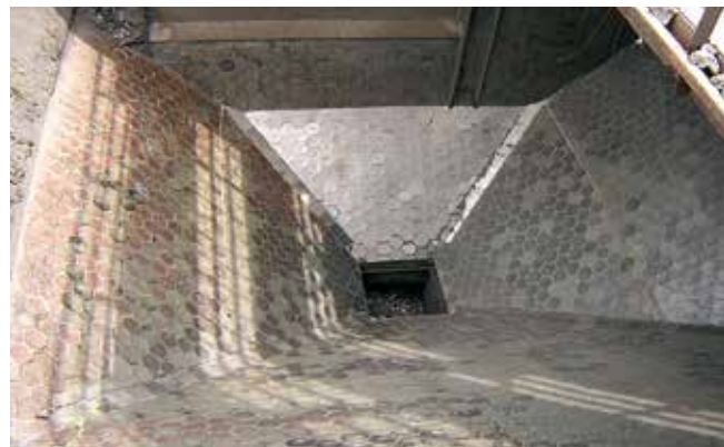
Proven wear protection material for bunkers in the coke handling is ABRESIST fused cast basalt
