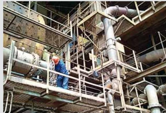
In Brazil the rubber lining in the pipe from the grinding mill to the classifying of the iron ore failed after a short time. These pipes are now lined with KALCOR zirconium corundum.
