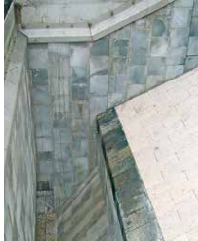
A trouble-free material flow is ensured in coal bunkers by the use of KALEN slide promotion plastics
