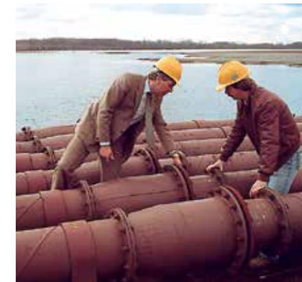
Long pipes require the use of expansion joints for linear extension.
