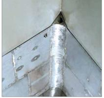
Apart from the lining itself, structural changes (e.g. angle of slope) mostly result in better flow properties. Kalenborn can offer complete solutions.
