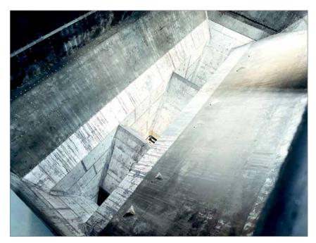
Slide promoting lining combination in the lower part of a high-level storage bin: fitted with KALEN linings on the inclined surfaces and KALINOX within the outlets which are subject to more intense wear.
