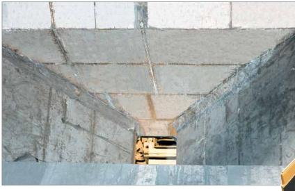
KALINOX linings will restore proper functioning even of older bunker systems.
