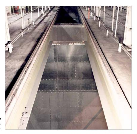
KALEN lining installed in a large German coal-fired power station. The material in the bunker is fine coal.
