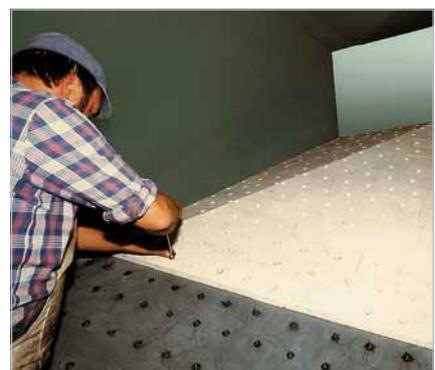
Mechanical fixing to meet special requirements
