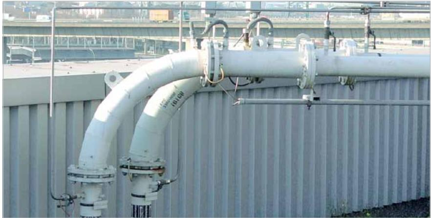
KALDETECT installed in a German waste incineration plant
