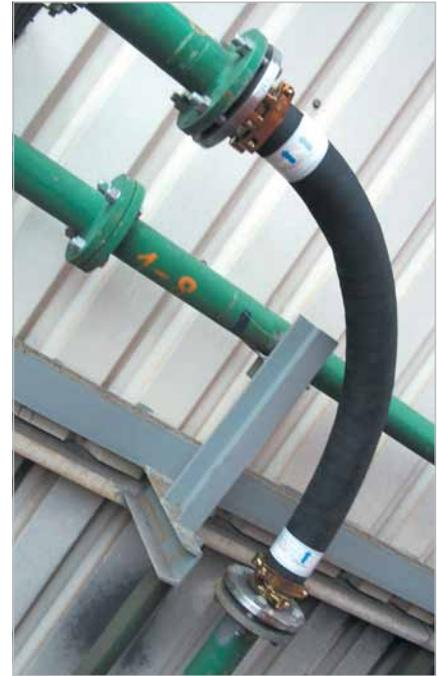
KALFLEX used as flexible pipe bend
