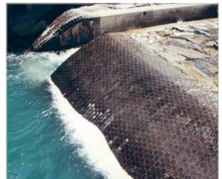
Irrigation wear protected by ABRESIST
