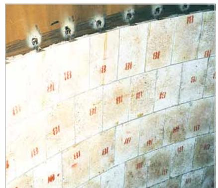
High temperature wear protection in a dedusting cyclone of a blast furnace plant in Europe
