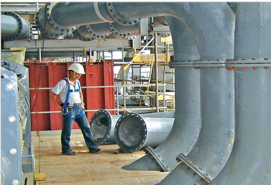
Typical applications of KALMETALL-C hard casting are pipe systems; here a pulverized coal pipe of a power station in South East Asia
