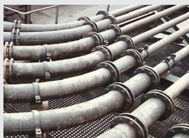
To reduce the severe abrasion of the bends in pneumatic systems, abrasion resistant piping components with internal linings – such as ABRESIST – should be used.
