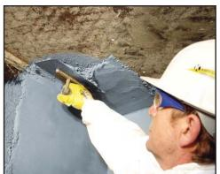
KALPOXY® NS is a non-sagging epoxy bonded wear compound designed to solve wear and abrasion on almost any surface. It contains ultra-high loading levels of silicon carbide (70%) and is mixed with DuPont Kevlar® fibers to create a unique non-sagging epoxy bonded wear compound with exceptional abrasion resistance and toughness.
