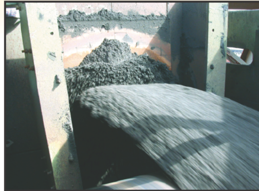
KALIMPACT installed at a ship unloading facility handling taconite
