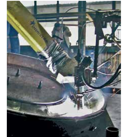
Kalenborn Service solves wear problems on site
