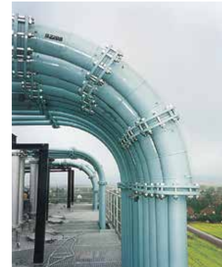
Protection for pneumatic and hydraulic pipes
