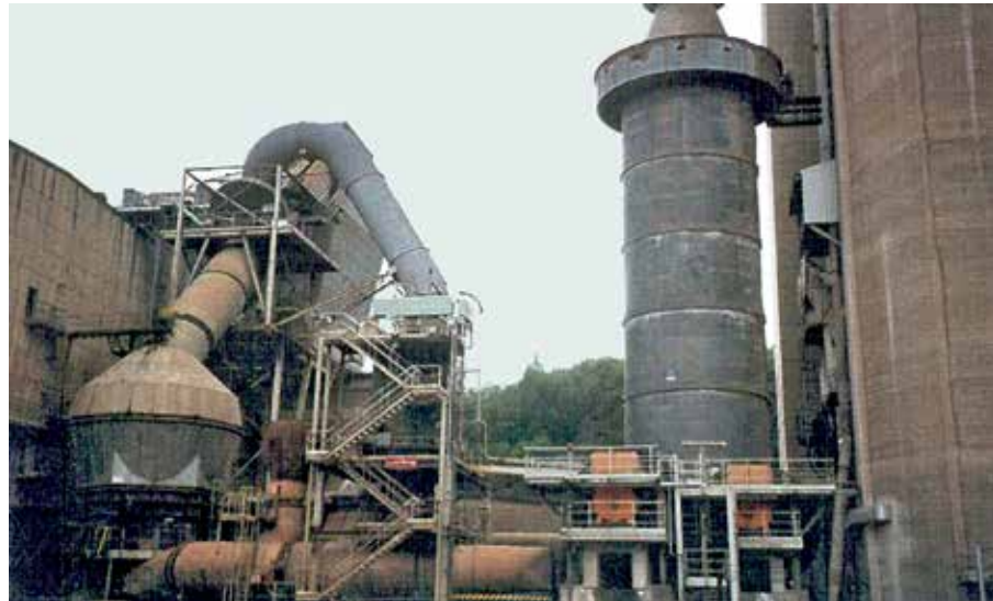
Reliable protection of raw mill and duct system with KALCRET BNX hard compound
