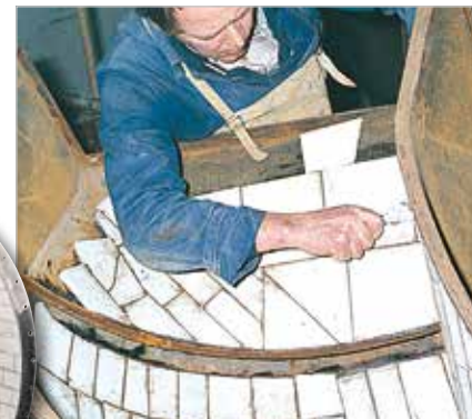
Chutes lined with KALCERAM are a solution that lasts, e.g. for bag loading systems in cement plants
