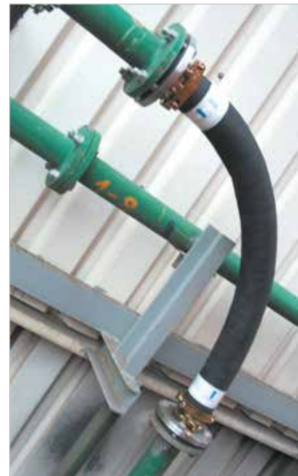
KALFLEX used as flexible pipe bend
