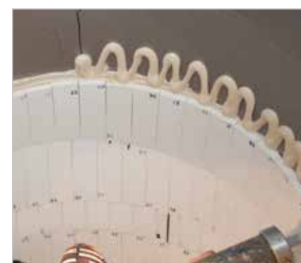
Lining with KALOCER mosaic mats in KALFIX setting compound
