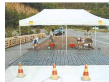
ABRESIST has performed well on automobile test tracks all over the world. Here, skid tiles are laid in Switzerland.
