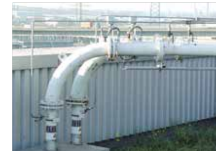
KALDETECT installed in a German waste incineration plant
