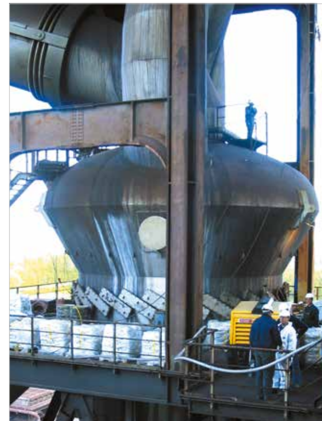
Scrubber inlet in a steel plant lined with sprayed-on KALCRET hard compound
