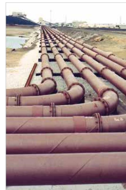
Worldwide ash removal pipes lined with ABRESIST reach lifetimes of more than 30 years. This US power plant operates more than 10,000 meters of 294 mm ID pipes.
