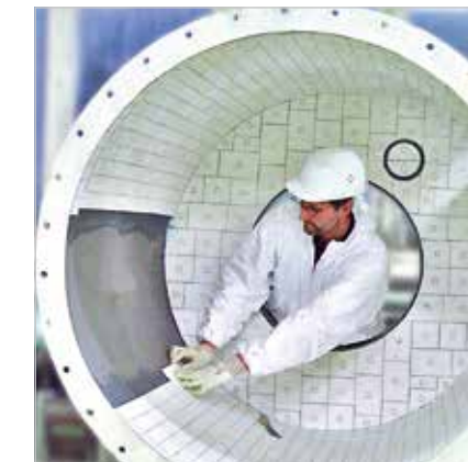
Lining a cyclone inlet with KALOCER; the vaulted form makes it possible to fix radial shaped elements in KALFIX setting compound whereas the headwall requires mechanical fixing by means of weld sleeves and ceramic caps.
