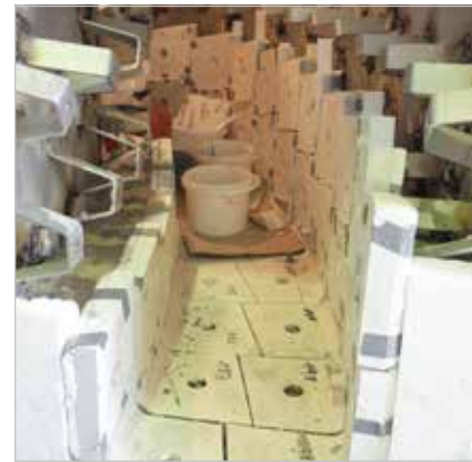
Convex dryer in a petrochemical plant with KALCOR
