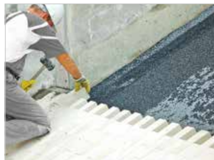
High temperature KALCERAM chute in a coking plant provides good sliding properties even at high temperatures
