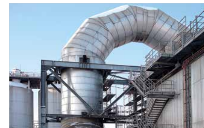
Clinker dust line in cement plant
