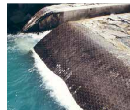
Irrigation weir protected by ABRESIST
