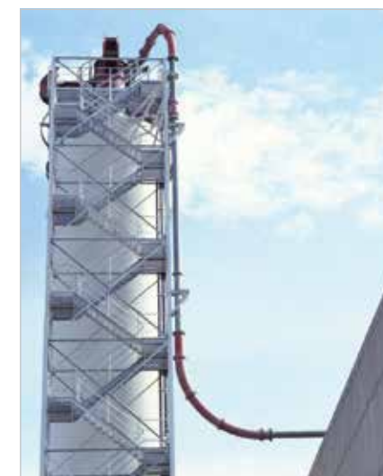
The bends and straight extension sections of the feed pipes to cement silos have been lined with ABRESIST
