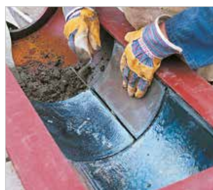
Setting in cement mortar
