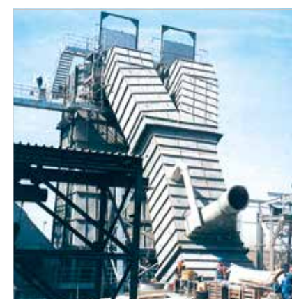
Reliable protection of the dust collecting pipe of a clinker cooler with KALCRET fitted as prefabricated shaped elements with integrated insulation
