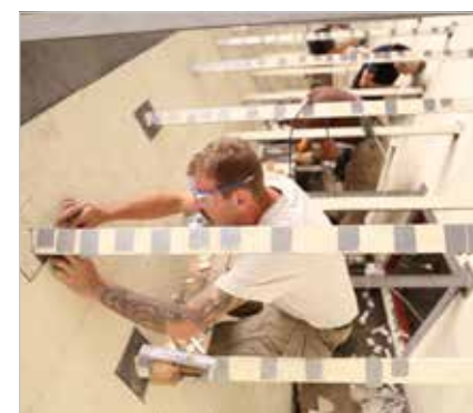
Lining with KALOCER mosaic mats in KALFIX setting compound
