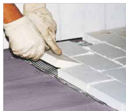
Lining and fixing with synthetic resin putties
