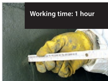
4. Check layer thickness and equalize it, if necessary
