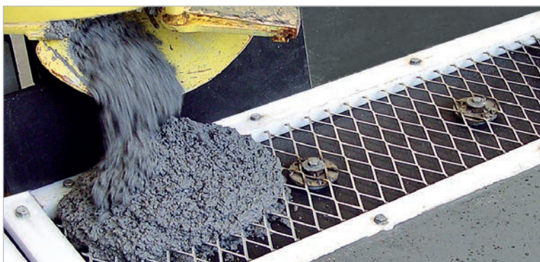
5. The compound should have a plastic consistency
