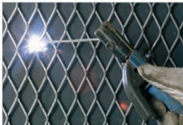
Welding the wire mesh to the surface: spacing approx. 250 mm / 9.84 inches
