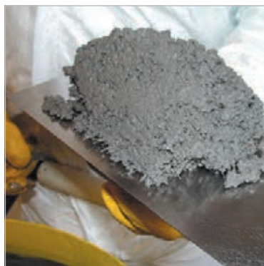
6. The stiff / plastic KALCRET compound (X) to be applied by trowelling with the aid of simple bricklayer tools
