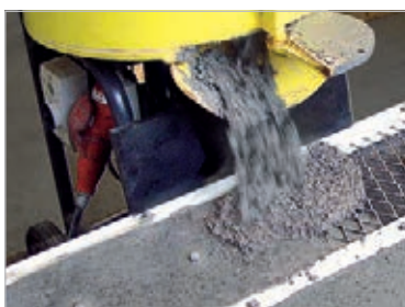
3. Carefully fill formwork
