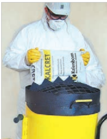
Material feeding into the forced circulation mixer
