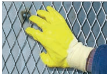
Stiff and rigid fastening – distance to the wall to be lined: about 5 mm / 0.19 inches
