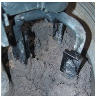
5. The compound should have a stiff / plastic consistency
