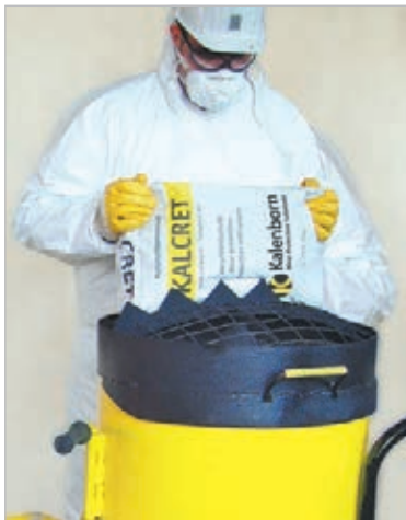
Material feeding into the forced circulation mixer
